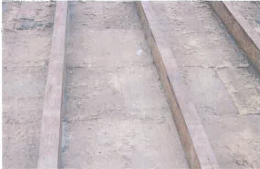
Photo no. 1, roof
