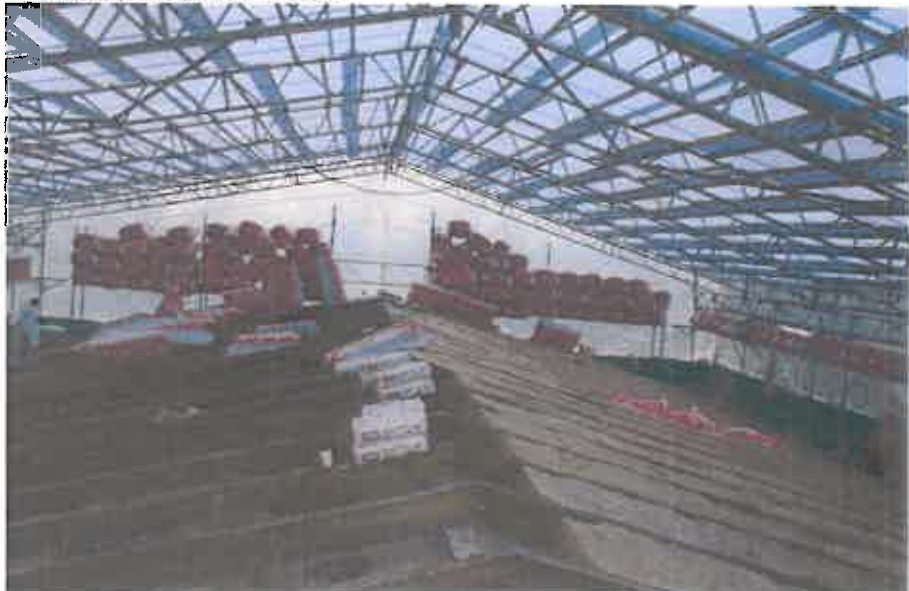
Photo no. 4, The construction site
